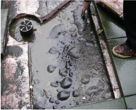
Typical Osmotic Blistering and Premature Failure of a Cold-Applied Waterproofing Membrane within an Inverted Roofing (PMR) Assembly over a Cast Concrete Slab
